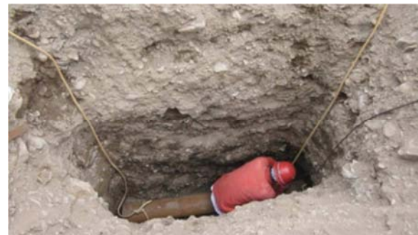
Figure 3. The high silicon cast iron auxiliary anode in the anode pit.
