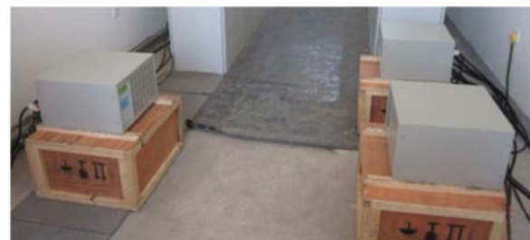
Figure 5. The constant potential rectifier of the temporary cathodic protect system.
