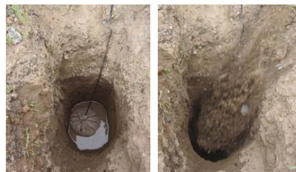
Figure 4. The construction process of burying the reference electrode.
